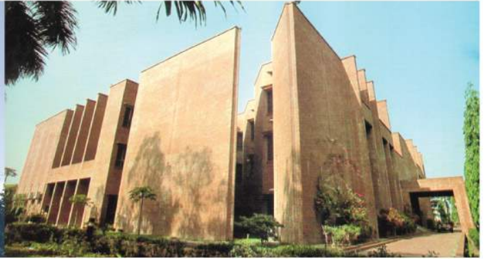
Bangladesh National Library and Archives Fire Detection & Alarming System
