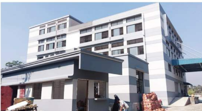
Berger Becker Bangladesh Limited Fire Doors, Fire Detection, Fire Hydrant, Fire Sprinkler, Public Address and Foam & FM200 Fire Suppression System
