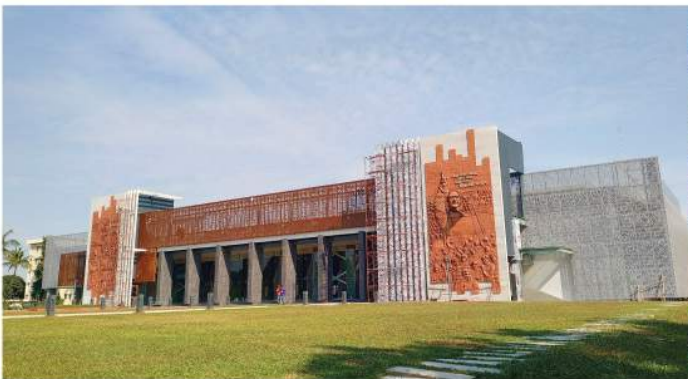
Senakunja Fire Hydrant and Fire Detection System
