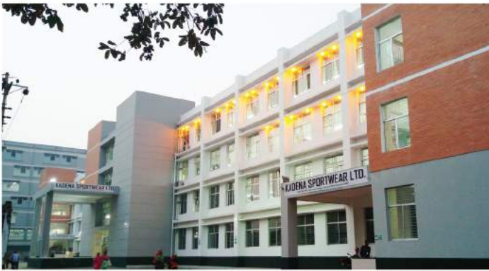
Kadena Sportswear Ltd. (Comilla EPZ) Fire Detection, Fire Doors & Protection System
