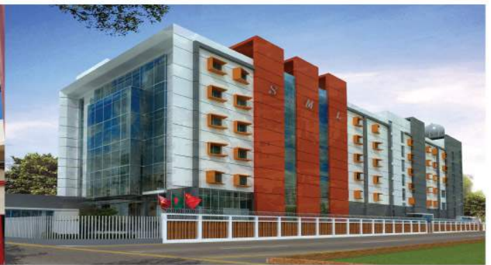
SML Packaging Solutions Bangladesh Ltd. Fire Detection, Fire Protection and Fire Doors
