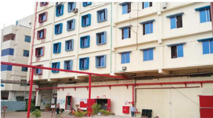
Loyal Apparels Ltd. Fire Doors, Fire Detection System & Fire Hydrant System
