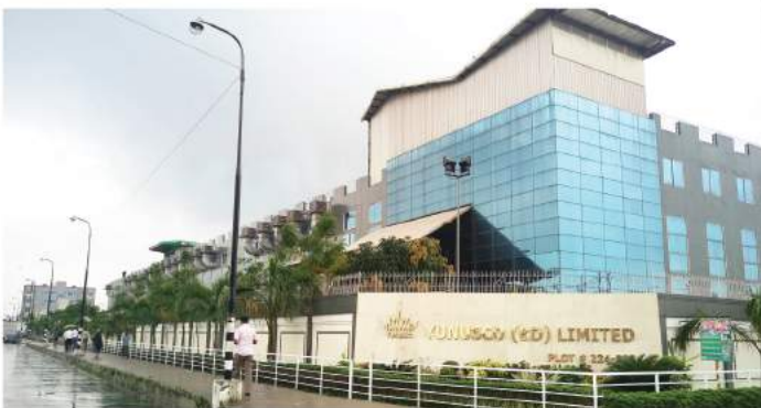
Yunusco (BD) Limited Fire Detection System and Fire Doors
