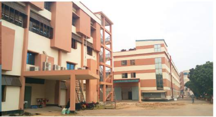
Lalmai Footwear Ltd. Fire Hydrant System (20 Sheds + 4 Buildings)
