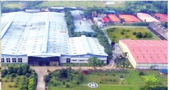
Partex Denim Ltd. Fire Detection System (Beam & Aspiration)
