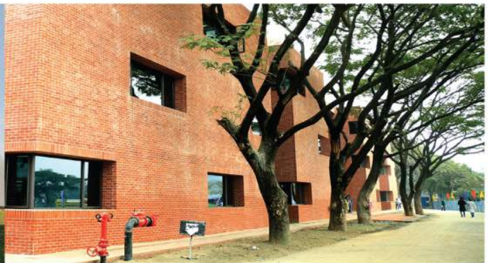
University of Liberal Arts Bangladesh (ULAB) Fire Detection & Fire Protection System
