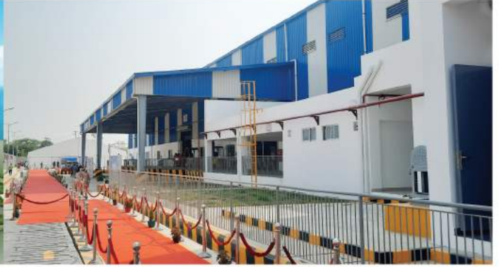
Berger Fosroc Ltd. Fire Detection System, Fire Protection System & Fire Doors
