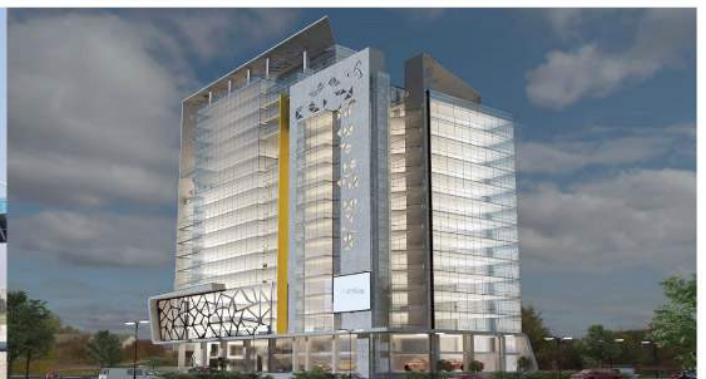
Rahman's Regnum Centre Fire Doors, Fire Detection, Fire Hydrant, Fire Sprinkler and Foam & FM200 Fire Suppression System
